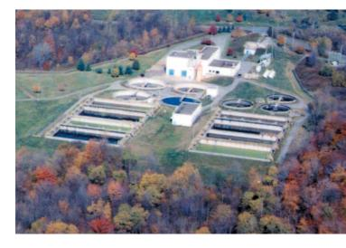
The plant is a conventional aerobic activated sludge design, with a reasonable amount of flexibility built in. Overall, the plant has run exceptionally well, and its operational costs were substantially below industry average. At the same time, the plant's environmental record was considered "unsurpassed" by any WWTP in the State of New York.
